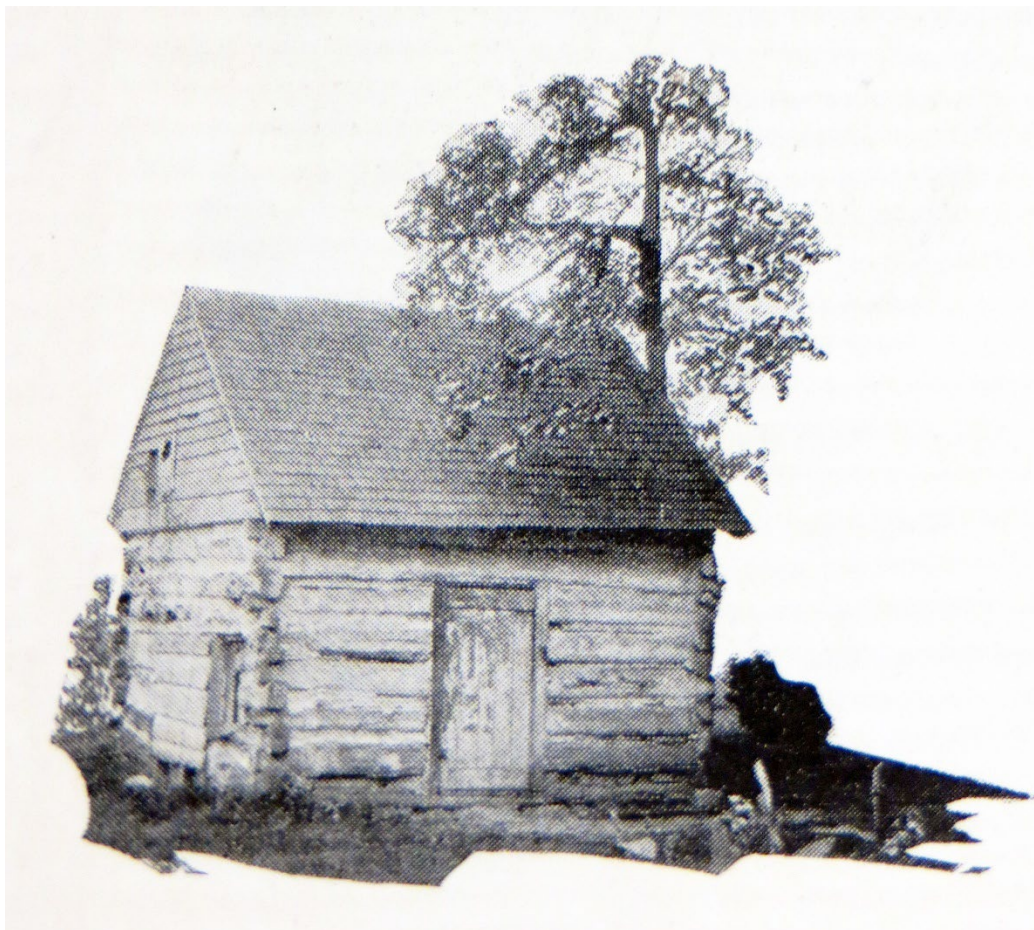
The log building, known as Rosati's Cabin
